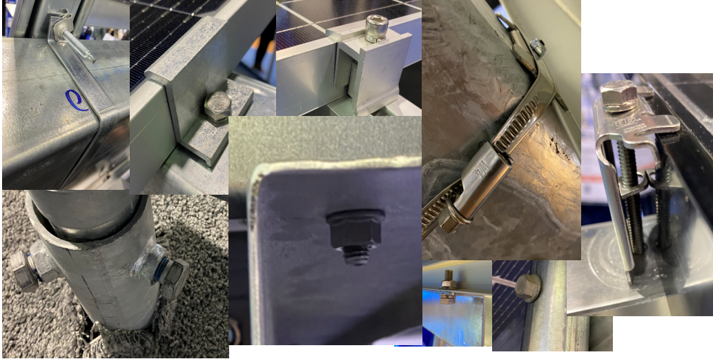
Figure 8. Alternative Structural Joints
