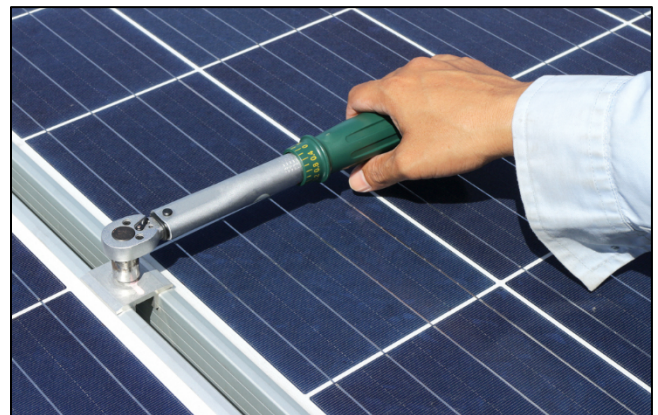
Figure 4: Example of an adjustable clicker-style torque wrench.
